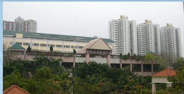
Shek Wu Hui Municipal service building
